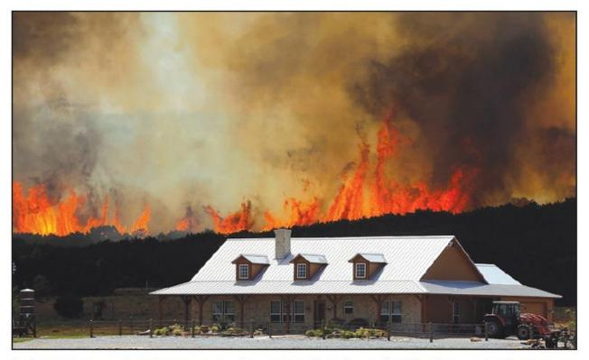
This home was constructed with fire-resistant materials — masonry siding and noncombustible roofing — and used Firewise landscaping practices that greatly increased its survivability and created a safer working environment for firefighters.
